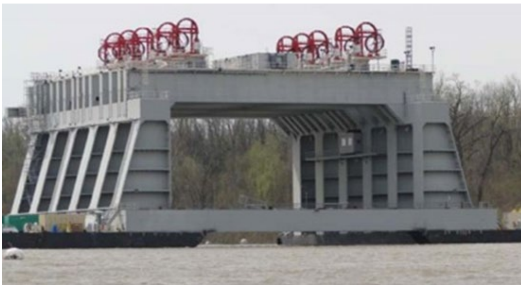
Figure 2. Catamaran Lift Barge
