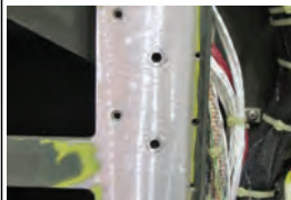
Patriot repair – wiring in proximity of repair
