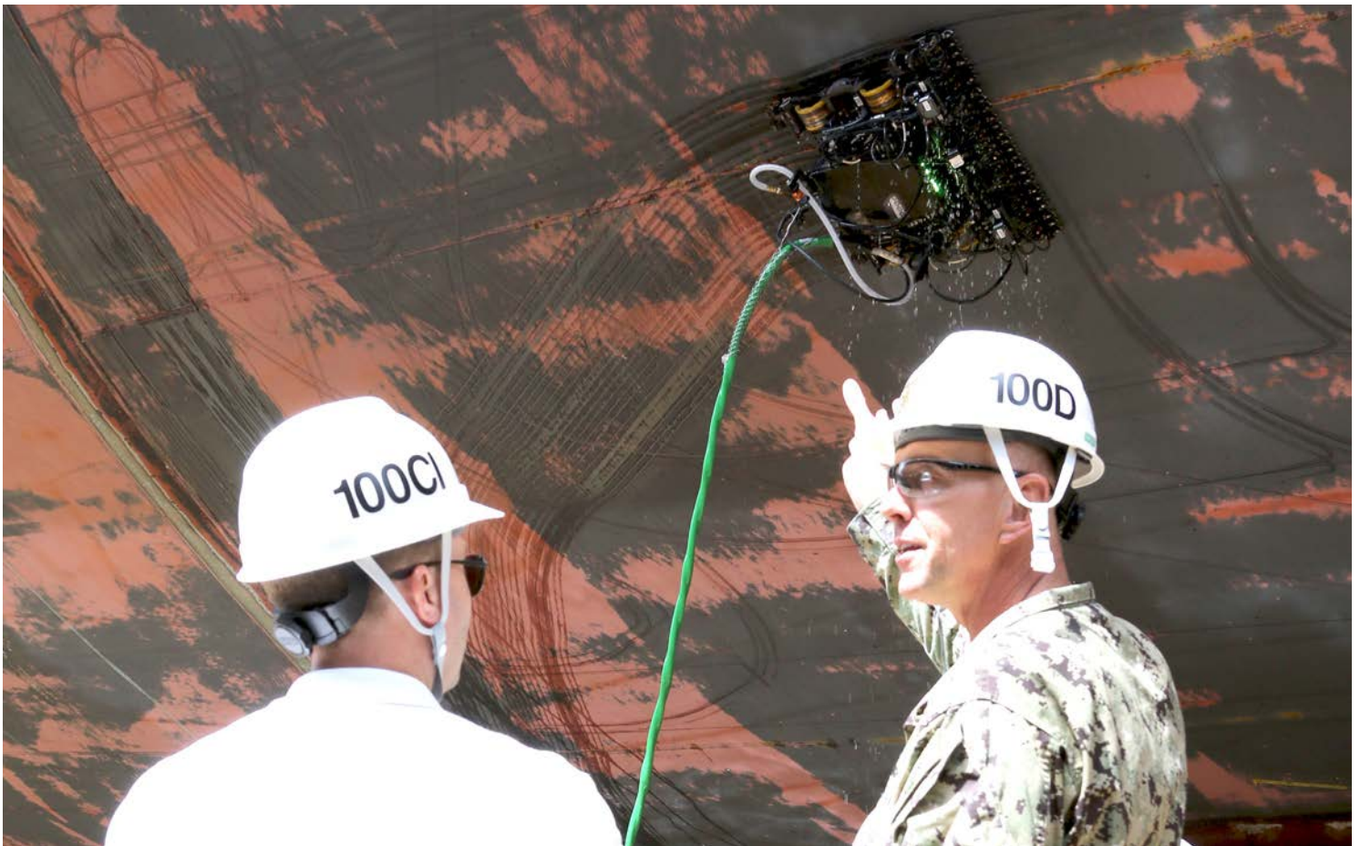
Demonstration of Gecko Robotics's TOKA wall-climbing ROV on the USS Howard while docked at the US Naval Ship Repair Facility and Japan Regional Maintenance Center in Yokosuka, Japan. (Photo courtesy of Japan Regional Maintenance Center Public Affairs Office.)
