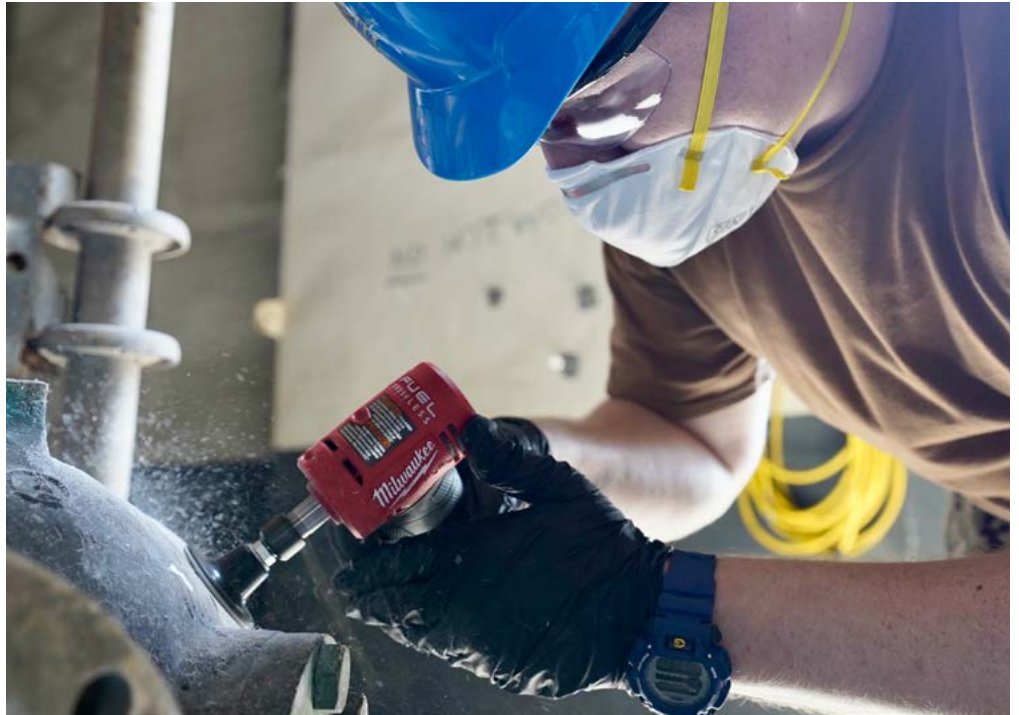
A Sailor sands off after epoxy repair on damaged equipment aboard the decommissioned amphibious assault ship USS Tarawa during the REPTX Salv-Ex event in May at PHNSY. (US Navy photo by Claudia LaMantia.)
