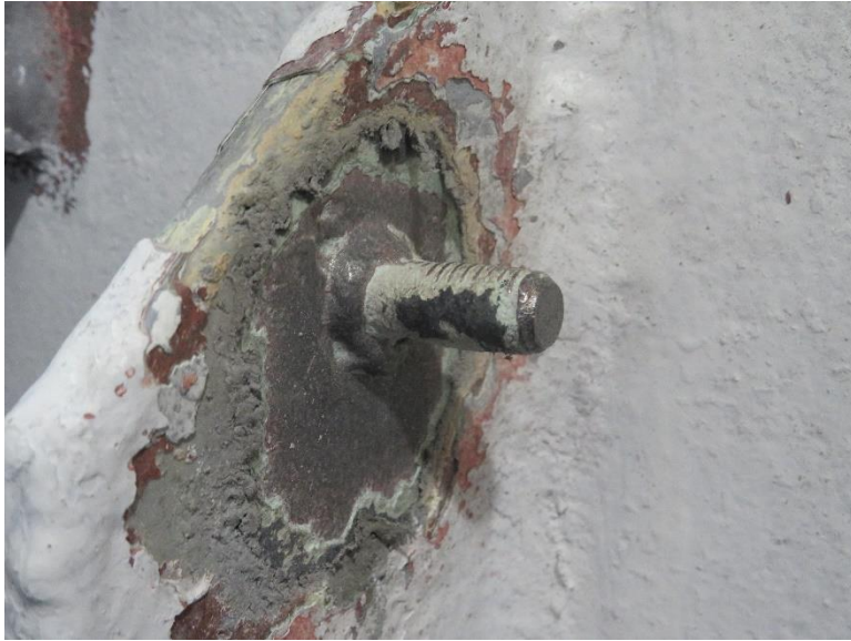
Figure 55: Sample Spot Sail-2-2 After Removal via Needle Gun March 13, 2020
