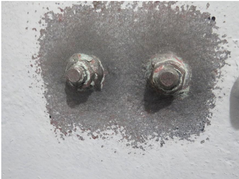
Figure 53: Sample Spot Sail-2-1 After Removal via Needle Gun. Underlying Surface Altered by Needle-Gunning Treatment March 13, 2020
