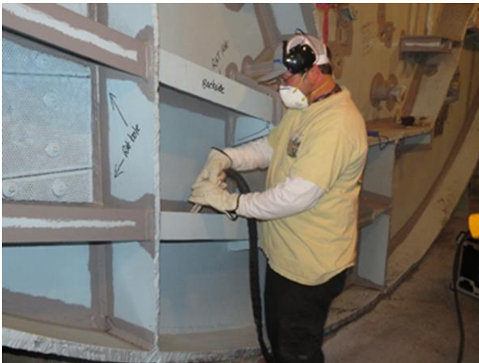
Figure 5. Application of APCR on Complex Geometry of Disused Submarine Section
