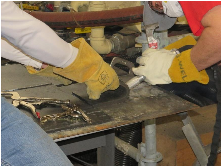
Figure 65: Sample Tile 4-B-5 Being Removed via Flensing with the PB7000M Tool March 11, 2020
