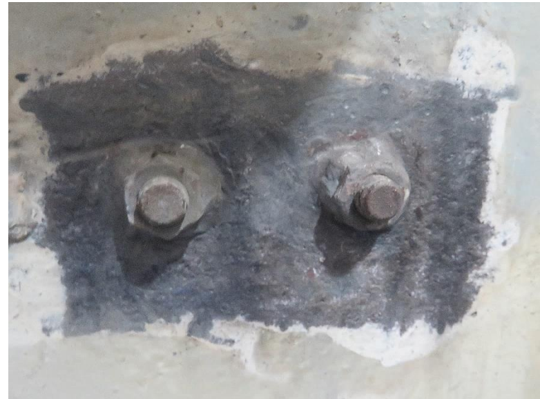
Figure 54: Sample Spot Sail-1-1 After APCR Treatment. Underlying Surface Revealed March 13, 2020
