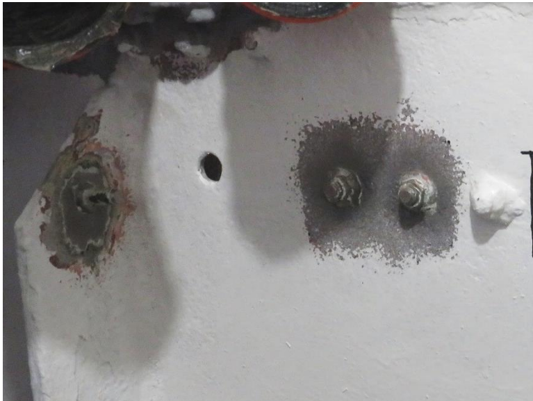
Figure 57: Sample Spots Sail-2 After Needle Gun Treatment March 13, 2020
