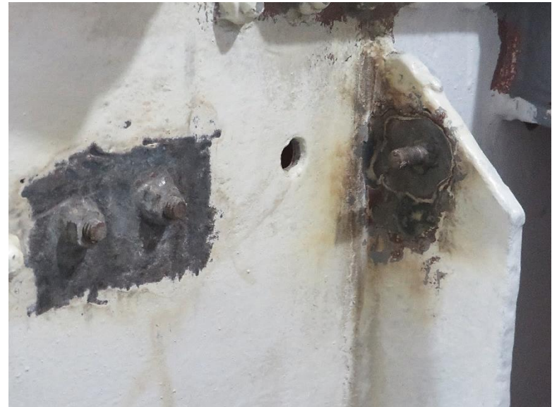
Figure 58: Sample Spots Sail-1 After APCR Treatment March 13, 2020
