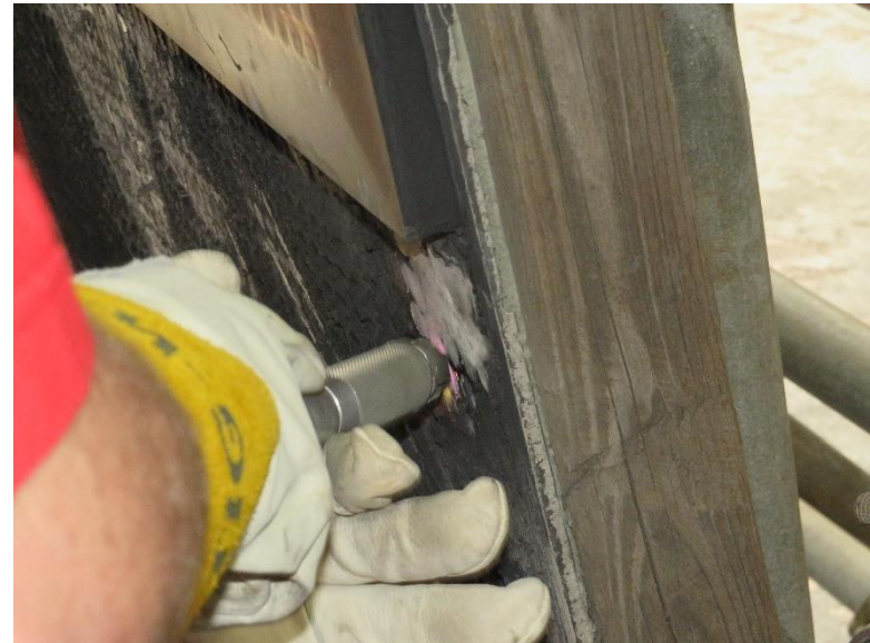
Figure 66: Leftover Honeycomb Tile Being Removed via APCR March 11, 2020
