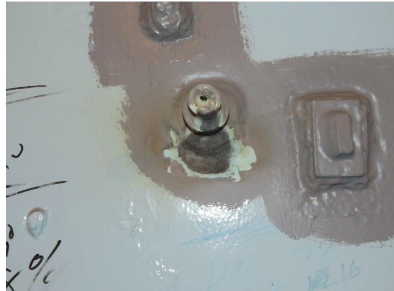
Figure 46: Welded Bolt Area Used for APCR Practice March 12, 2020
