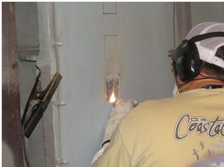
Figure 39: Sample Spot 17-1-Bottom Being Removed Via APCR March 12, 2020
