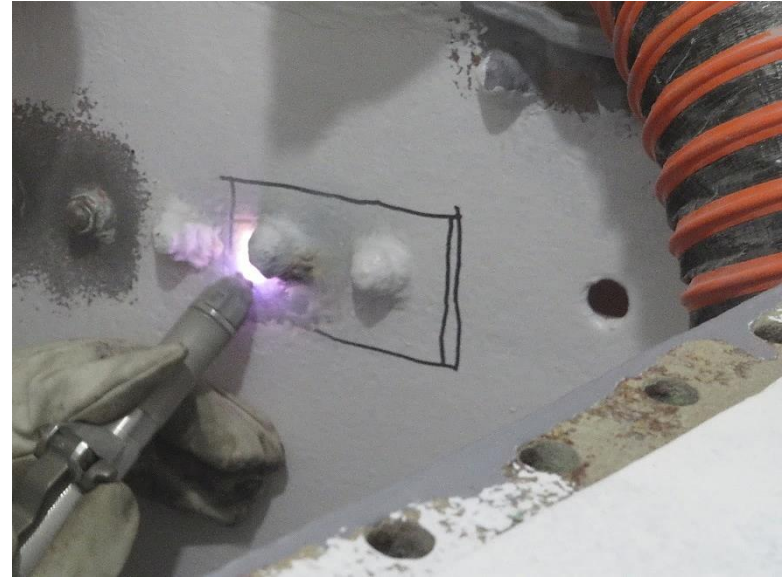
Figure 52: Sample Spot Sail-1-1 Being Treated with APCR March 13, 2020
