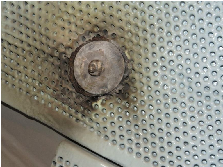
Figure 45: Sample Spot 18-3 After APCR Treatment March 12, 2020
