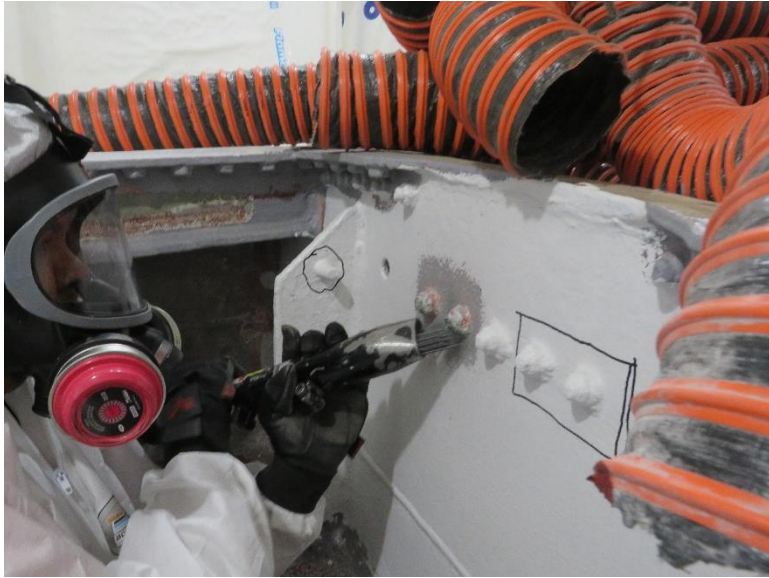
Figure 51: Sample Spot Sail-2-1 Being Treated with Needle Gun Scaler March 13, 2020
