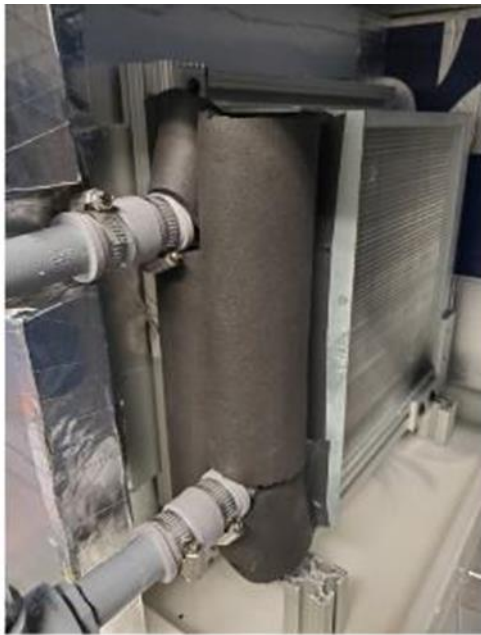
Figure 22. Glycol Supply and Return Hoses Penetrating into Plenum and Connected to Heat Exchanger
