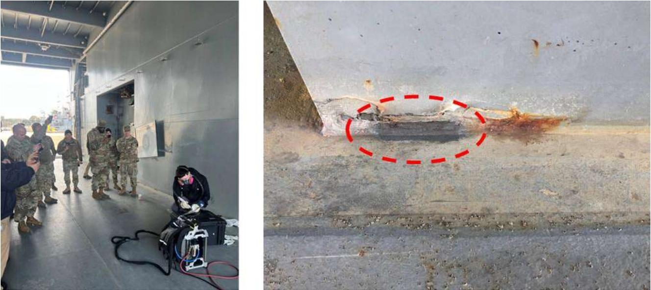
**Figure 3. Demonstration of PlasmaBlast 7000-M Technology to Army Personnel (left); Removal of Coating and Light-Corrosion Aboard LSV-1 (right)**
