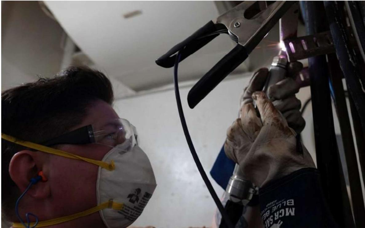
*Figure 2. Navy Maintainer Performing Coating Removal Aboard Decommissioned USS Tarawa*
