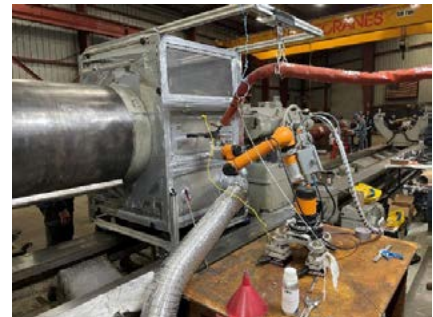
Pier-Side Rudder Stock Repair
