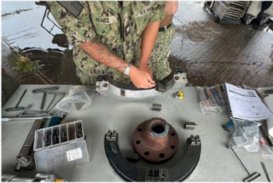
Trained U.S. Navy on the use of field machining equipment for battle preparedness exercise.
